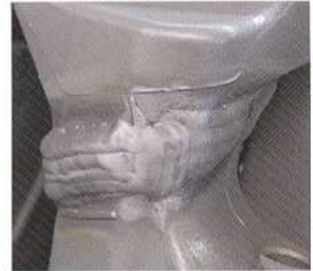
Welding beads with no wash applied.
